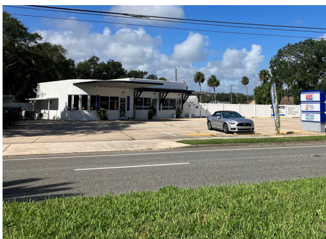
CRA Small-Scale CFPI Grantee: JARS Holding New Smyrna, Inc. 646 N Dixie Fwy- After Improvements (2021)
