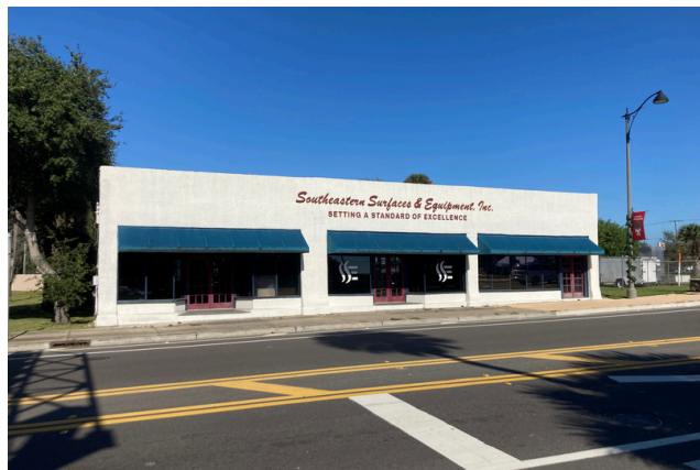
CRA Small Scale CFPI Grantee: SSE & Associates, Inc. 569 Canal St.-Before Improvements (2022)
